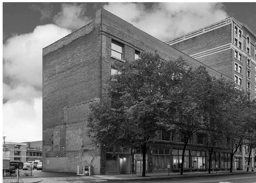
#1104 in 2024 is the second entrance from the left.
